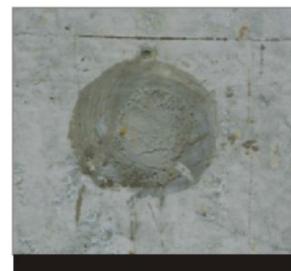
Patch the "Hole" by Non-Shrink Grout or Mortar Trám lỗ ty bằng vữa không co ngót - NS Grout
